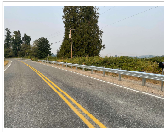
Mud Lake Road Guardrail
